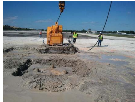
Fig. 20 1 st tamping (Lot of water comes up)
