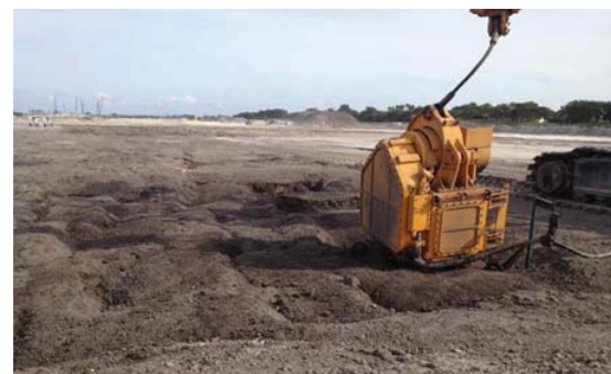
Fig. 21 2 nd tamping (No water comes up)
